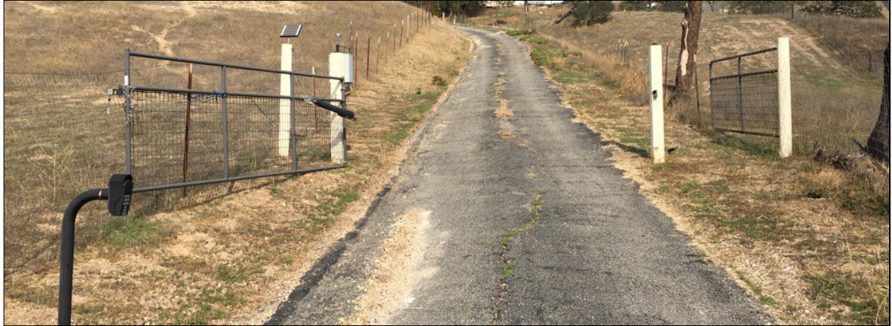
Figure 6.1.1 Gate at the bottom of the PFH driveway.
