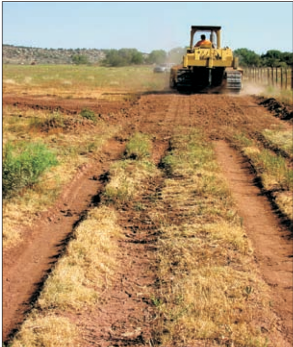
Photo V-10: Tractor constructing reverse slope ramp beyond lead-out ditch using the stockpiled fill (photo V-9).
