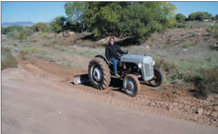
Photo IX-7: Antique farm tractor making a lead-out ditch with a scraper blade.
