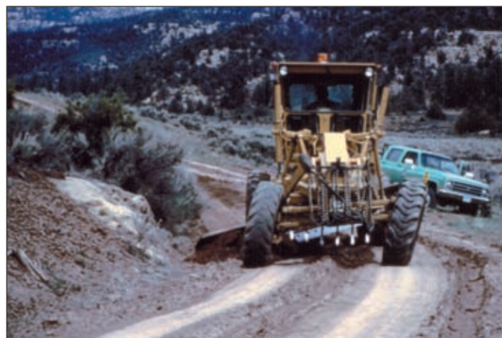
Photo V-3: Blading to maintain an insloped road template.
