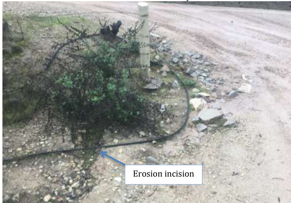
Figure 3-6 Erosion on south side of driveway entrance
