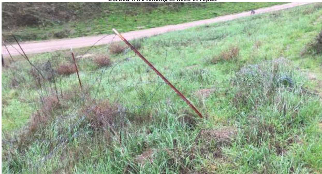
Figure 6-1 Barbed wire fencing in need of repair
