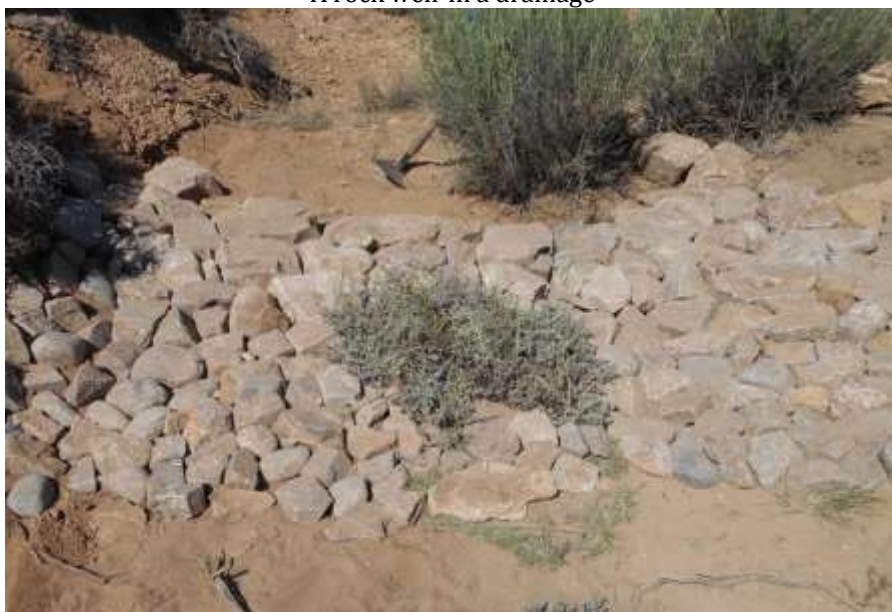
Figure 2-6 A rock weir in a drainage
