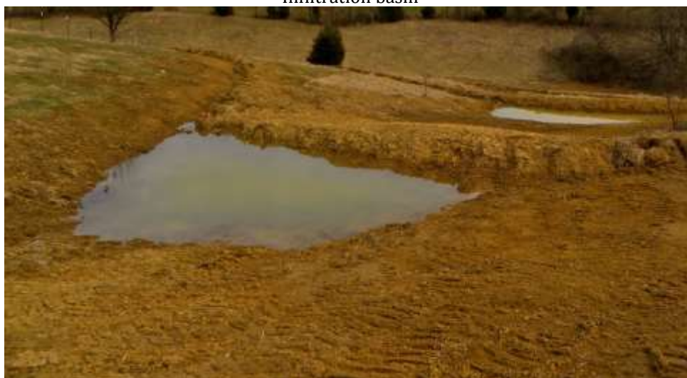
Figure 2-9 Infiltration basin
