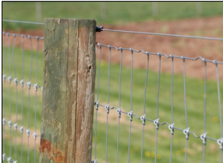
Figure 6.2.4 Woven wire fencing is recommended for animal enclosures as it can handle being pushed against by animals without welds breaking or being bent permanently out of shape.
