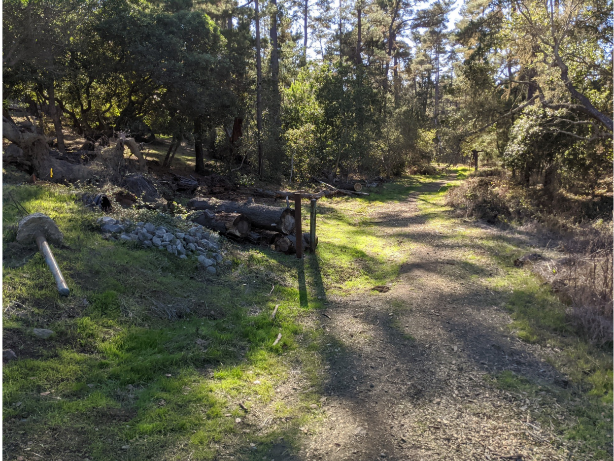
Figure 5: The outlet of second-highest culvert draining water across the portion of Burton Drive uphill of and that ultimately feeds onto the Greenspace Strawberry Canyon property. This culvert empties directly onto the Greenspace Strawberry Canyon property, where it pools on and drains down the utility access road shown. Photo taken from Burton Street.
