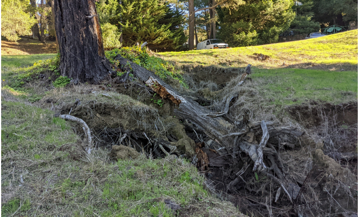
Figure 4: The headcut in the drainage channel just below of the outlet of the highest-elevation culvert located on the portion of Burton Drive uphill of and that ultimately feeds onto the Greenspace Strawberry Canyon property. The progress of which has temporarily arrested by the dead pine tree trunk.
